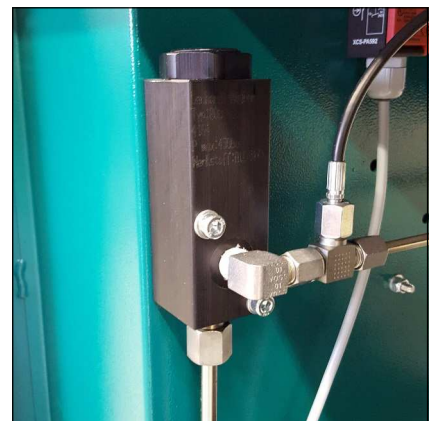
Pressure maintaining/non-return valve
