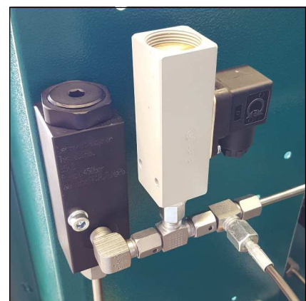
Pressure switch for start pressure
