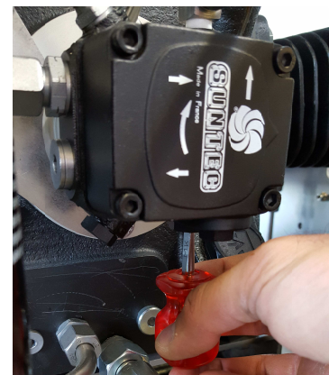
Adjusting the oil pressure
