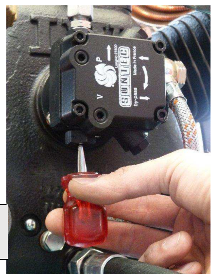
Adjusting the oil pressure
