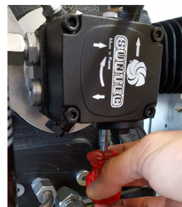
Adjusting the oil pressure
