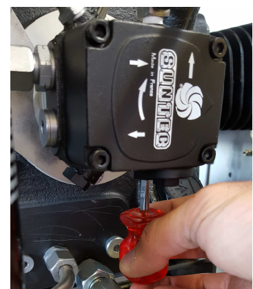
Adjusting the oil pressure
