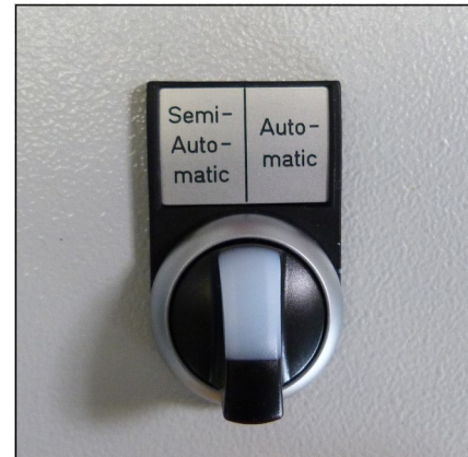
Selector switch auto start function
