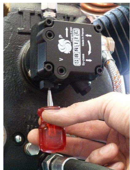
Adjusting the oil pressure
